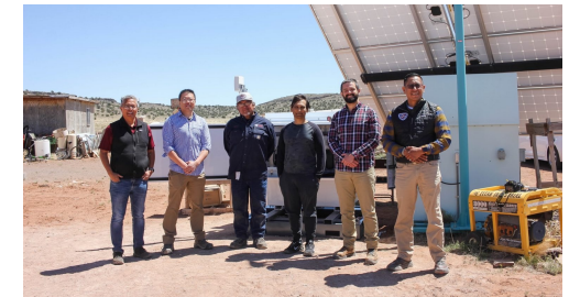
Urban Electric Power, Navajo Tribal Utility Authority, Sandia - ZnMnO 2 battery deployment
